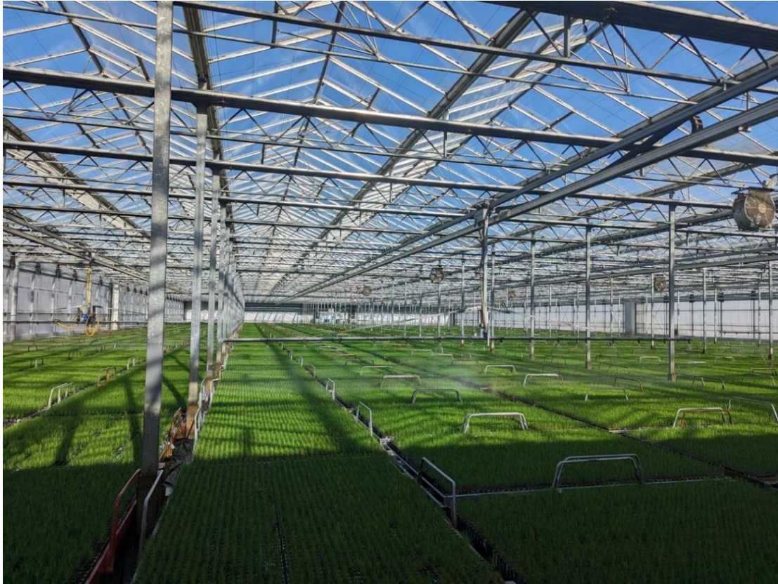
Figure 4 One of a number of greenhouses, with control, climate control and automated fertigation
