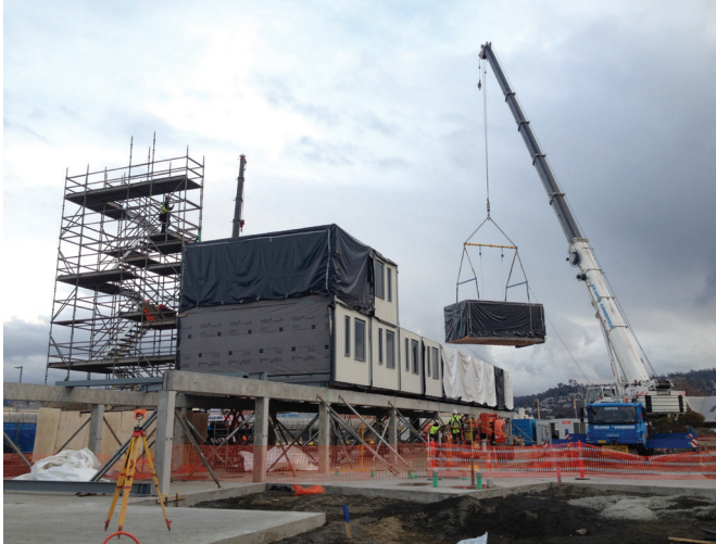
Figure 1 The Inveresk Apartments at University of Tasmania install prefabricated modular apartments. Image courtesy of University of Tasmania.
