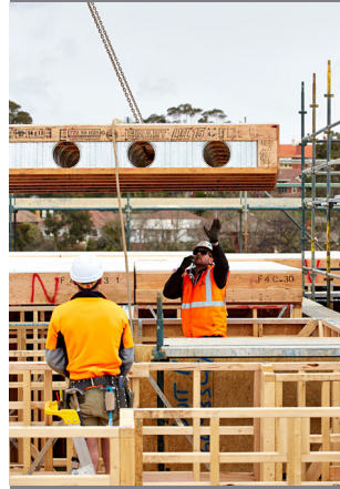
Figure 1 The Inveresk Apartments at University of Tasmania install prefabricated modular apartments. Image courtesy of University of Tasmania.
