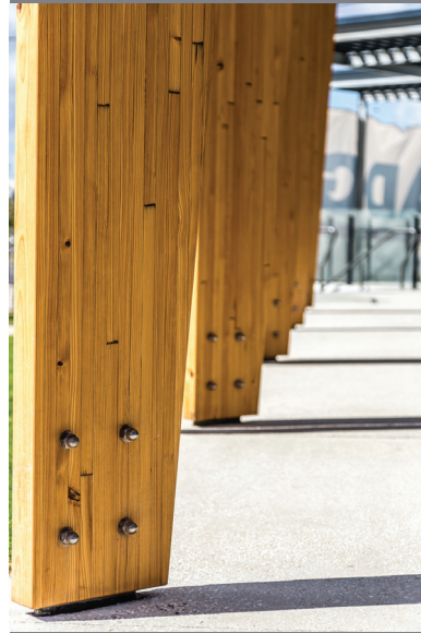
Figure 3. Glue laminated timber columns used in the construction of Stella Maris Church, Maroochydore. Image courtesy of Hyne Timber.
