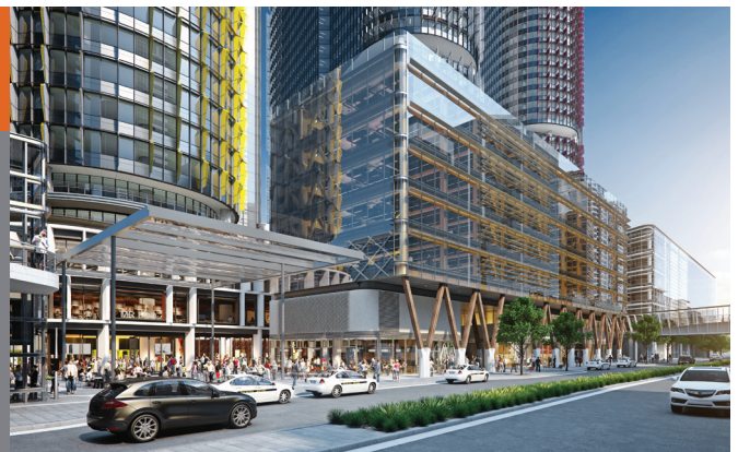
Figure 1 International House, Barangaroo, Sydney. Image courtesy of Lendlease.
