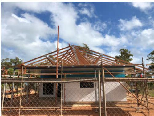
*Gumatj sawmill hardwood truss being used for local housing*
