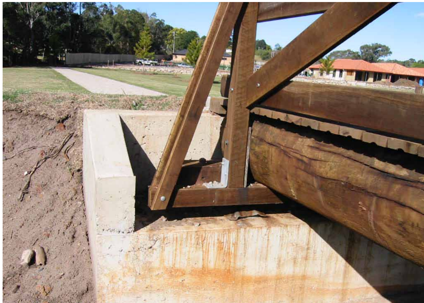
KFBRV Jetty - bridge head detail
