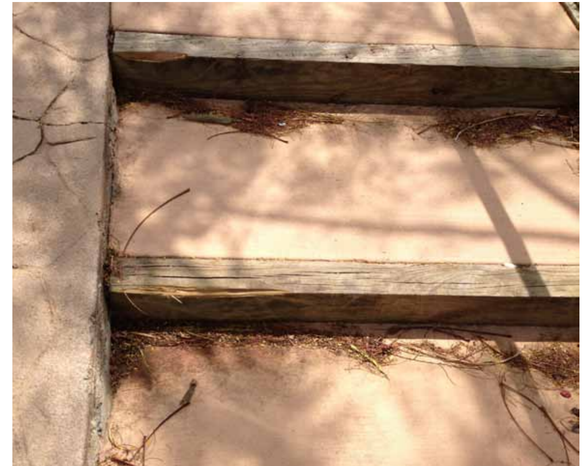
Concrete steps with hardwood timber sleeper ends / risers that are failing / warping (above).
