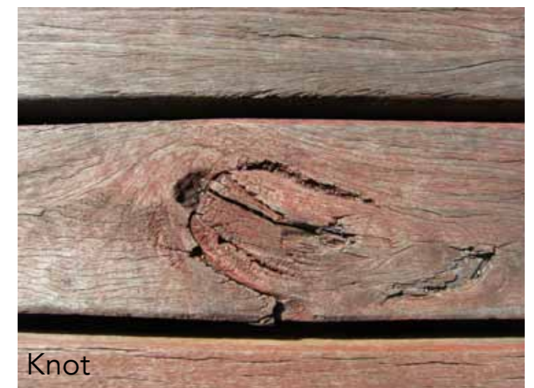
Examples of timber face imperfections
