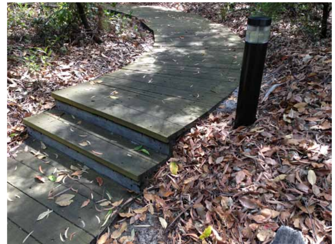
Concrete steps with hardwood timber sleeper ends / risers that are failing / warping (above).
