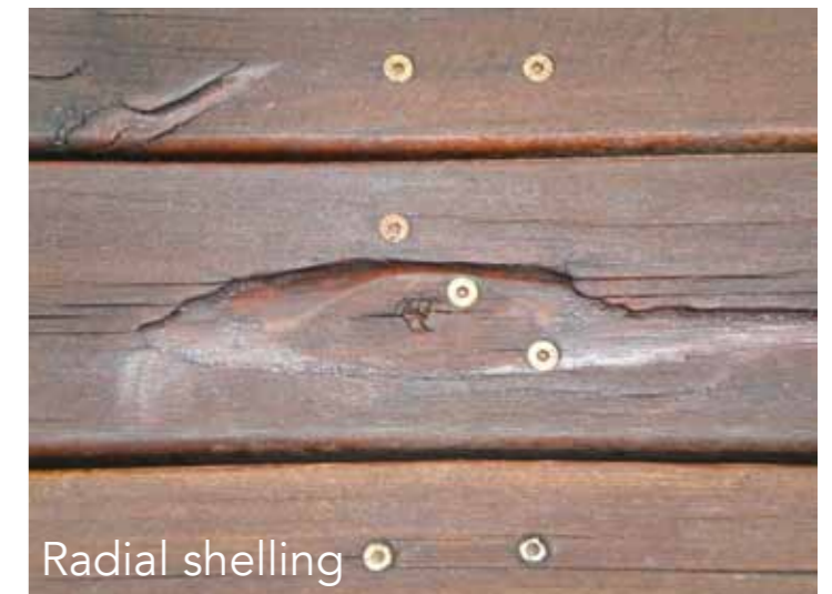
Examples of timber face imperfections
