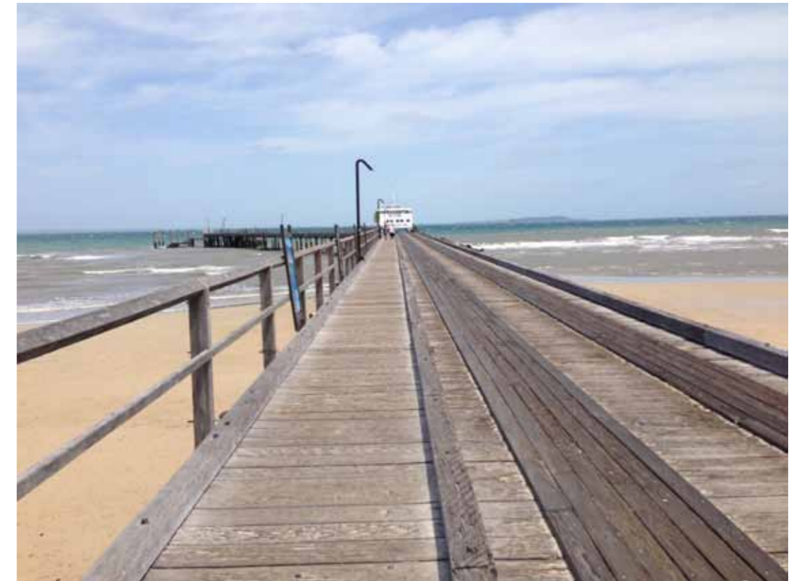
KFBRV Jetty - built 1989
