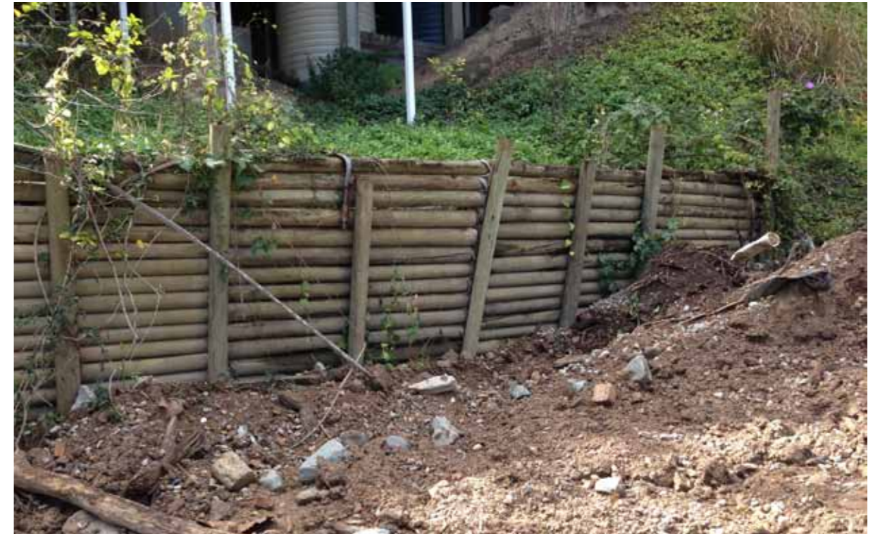
Failed CCA treated pine retaining wall (above). Raised timber sleeper garden bed at a school (below).
